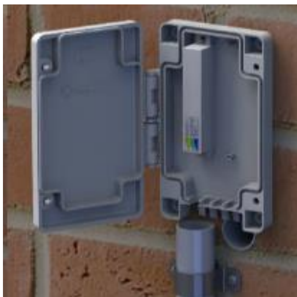
Figure 14. nbn NTD with VDSL2 centralised filter installed
