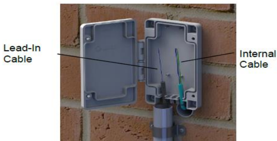
Figure 13. nbn with unterminated cables
